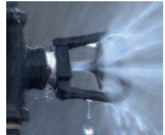
Right - Sprinklers prevent wide-spread fire damage.
